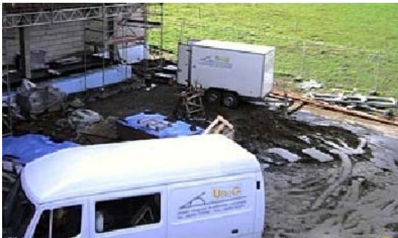
Figure 10: Original UBeG TRT-equipment of UBeG on site for design of a BHE field in Aachen, Germany
