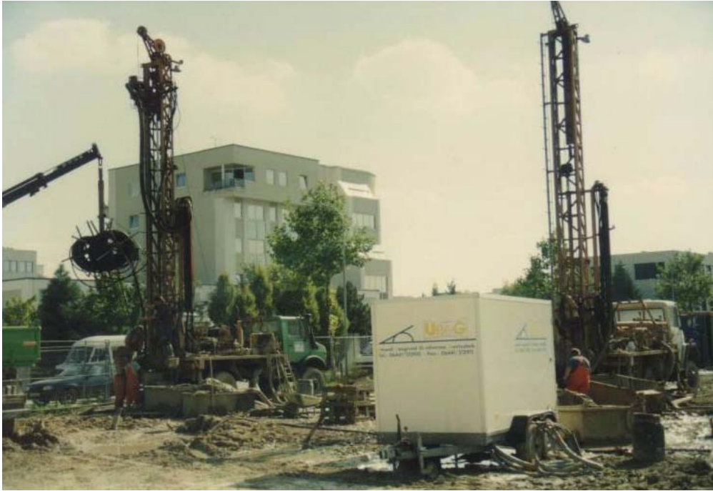
Fig. 8: Construction Site of Deutsche Flugsicherung, Langen, with borehole heat exchangers
